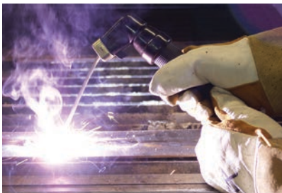
9) Hold the electrode slightly above the work maintaining the arc while travelling at an even speed.
