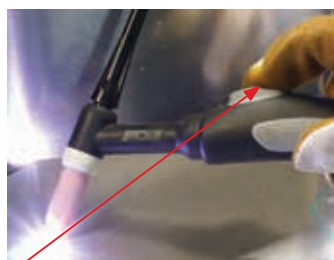
(5) Press the torch switch and the arc will ignite across the gap between the tungsten and work piece. Hold even distance of about 2mm gap between the tungsten and work piece to maintain the arc.
